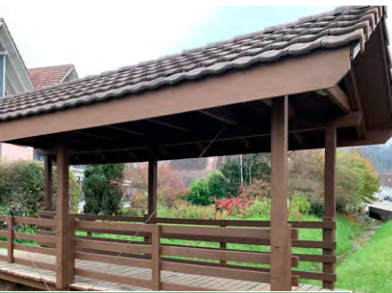
DORFBRÜCKE IN FELBEN-WELLHAUSEN
